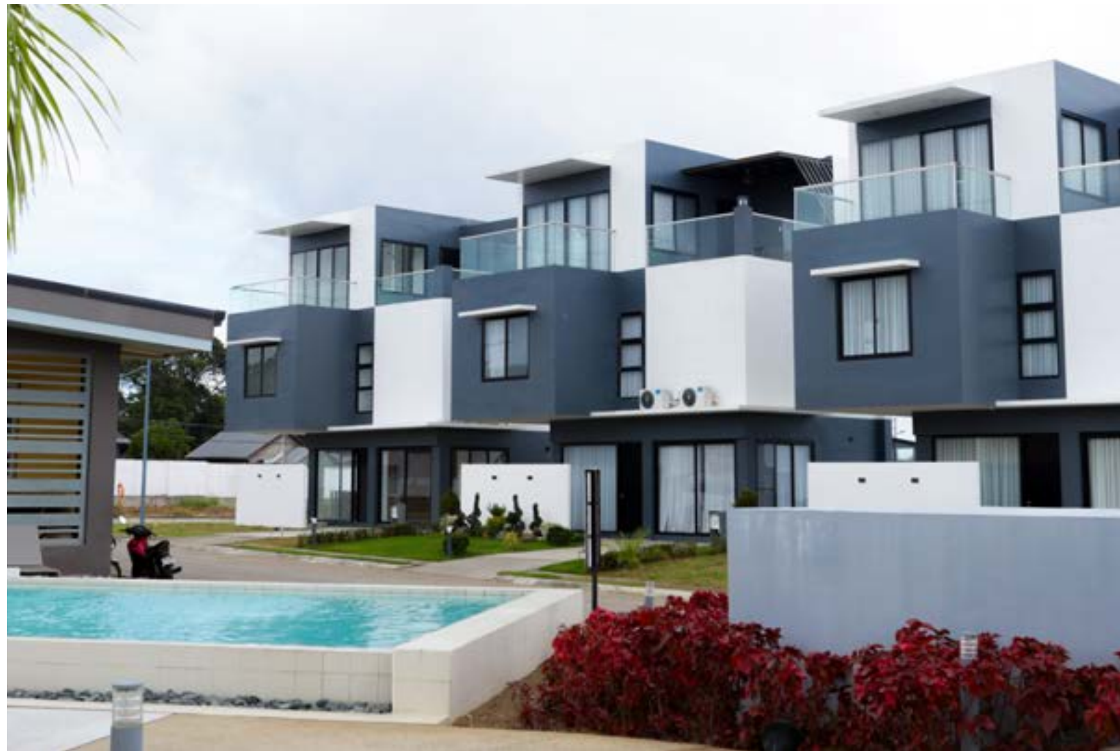
Completed Tranche Homes
