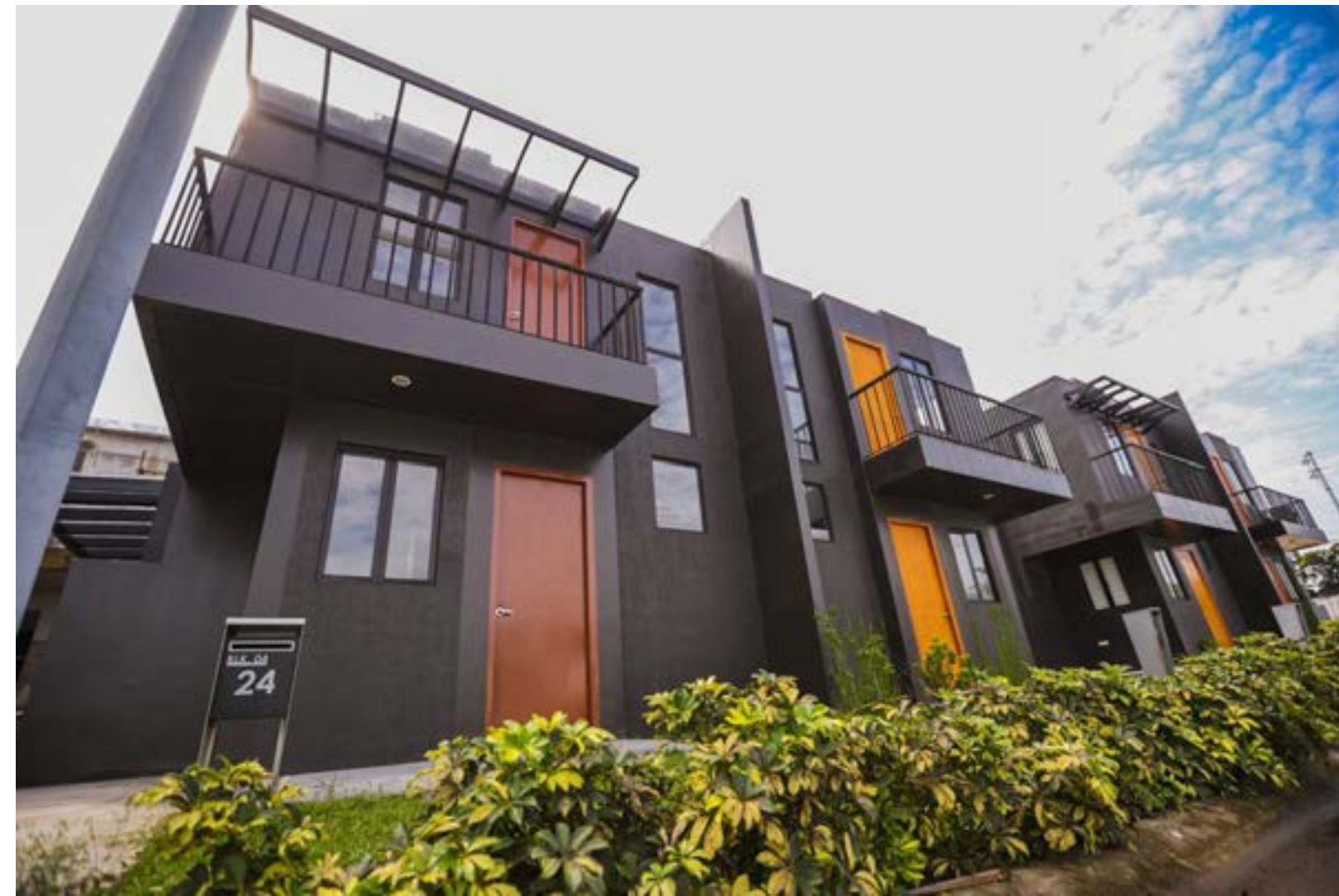
Completed Hedera Homes
