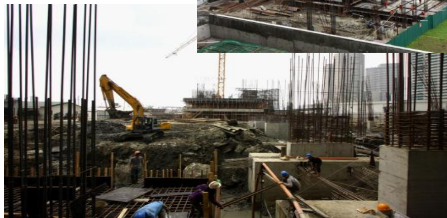
Dettifoss: column bar and shearwall installation
