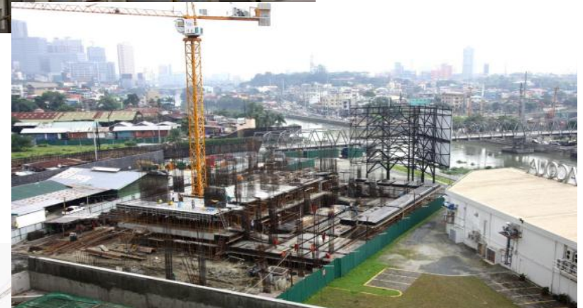
Livingstone: structural works for parking levels
