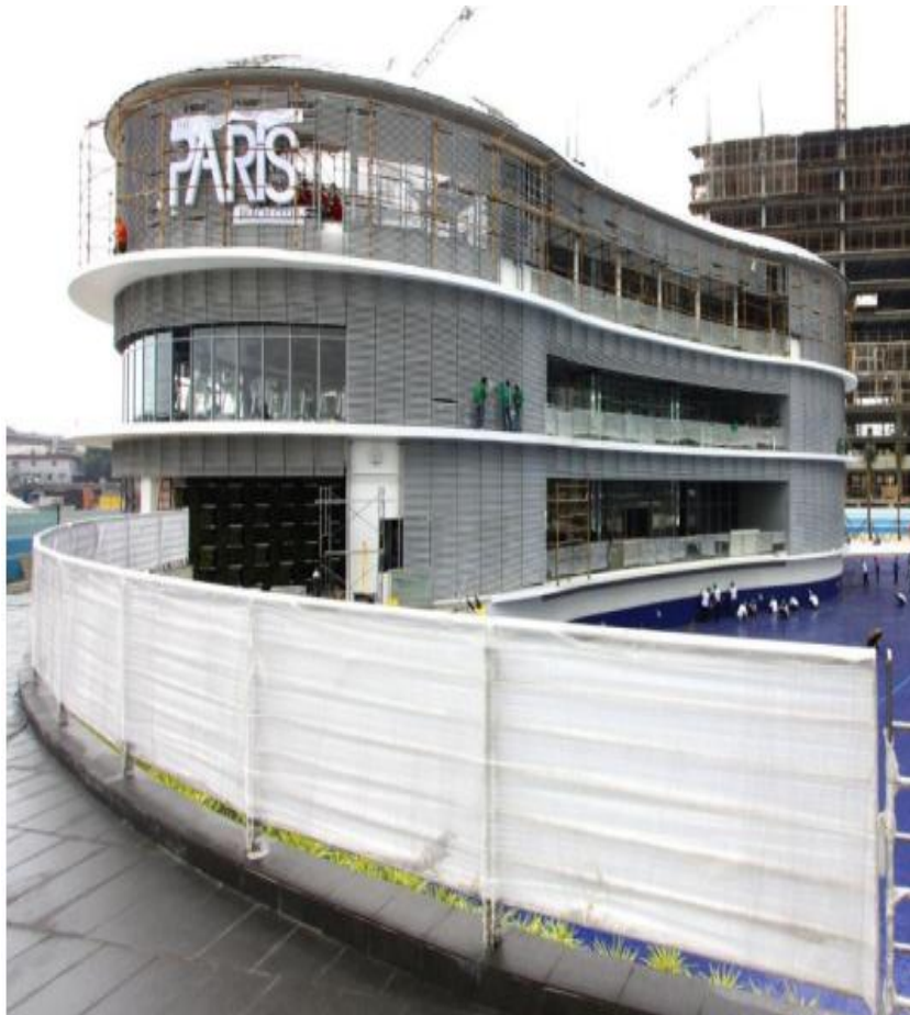
Paris Beach Club's exterior is almost complete with roofing works underway
