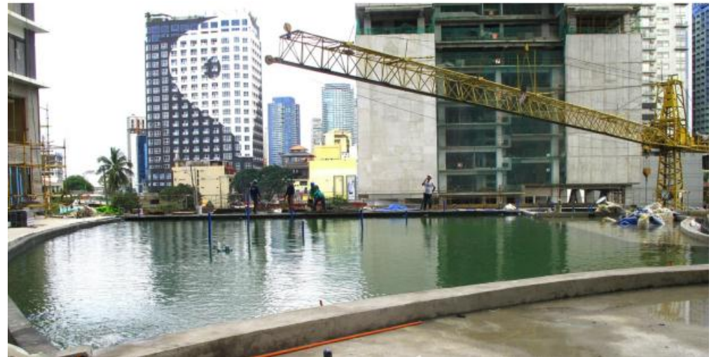
Waterproofing works for the Knightsbridge swimming pool are in-progress.
