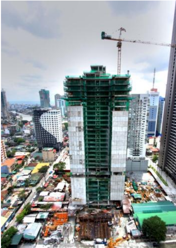
Centuria Medical Makati reached structural completion in September.
