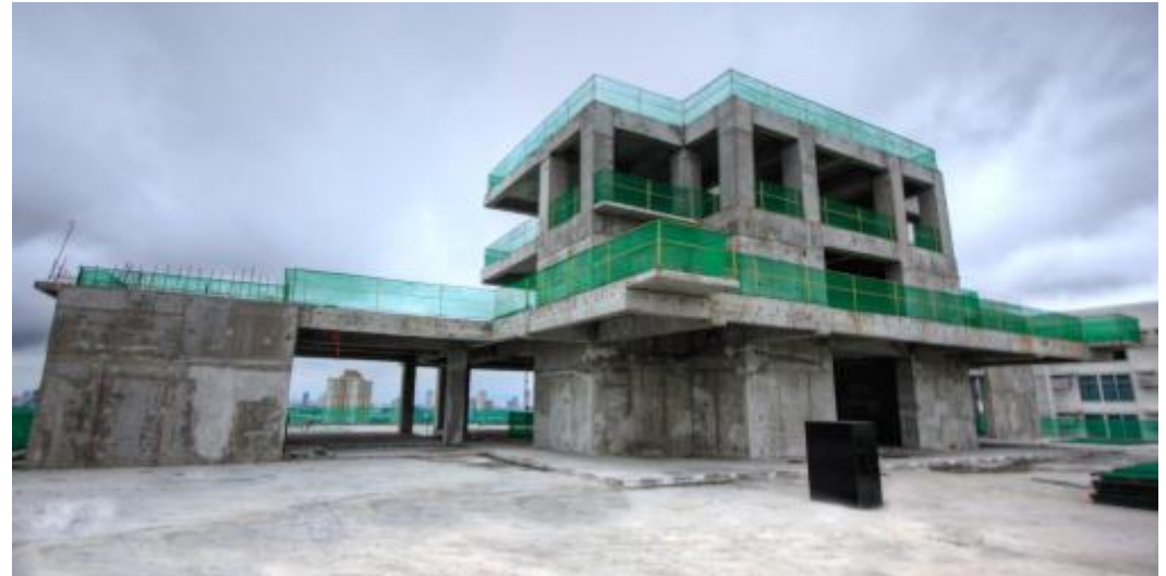
The roofdeck level of Centuria on the 28 th level
