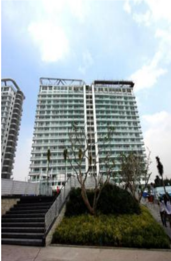
Azure's 3 rd tower, St. Tropez in its finishing stages
