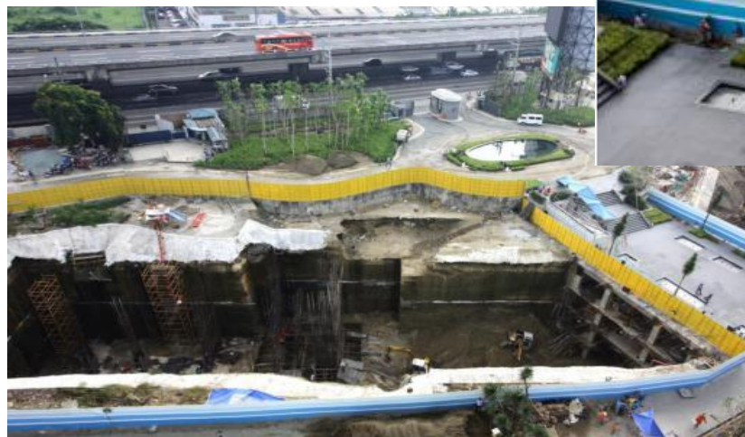
Boracay Tower undergoing formworks for its 4 th basement level
