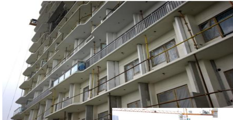
Niagara: Installation of balcony railings and windows
