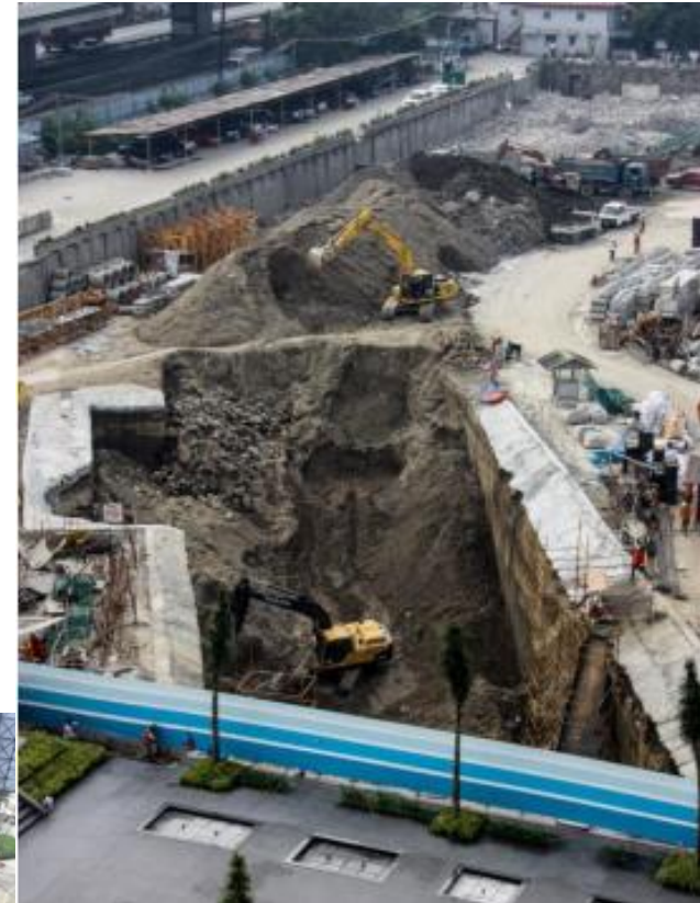
Site clearing works in full swing for Azure's 8 th tower, Maldives
