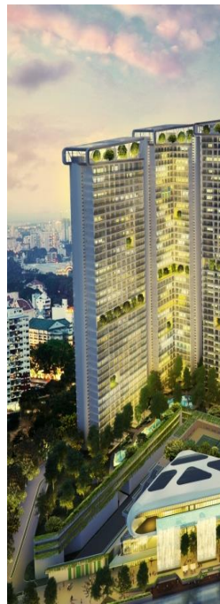
NIAGARA AT ACQUA COMPLETED IN FEB 2015
