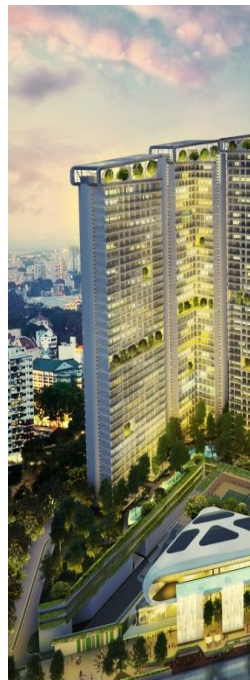
NIAGARA AT ACQUA COMPLETED IN FEB 2015
