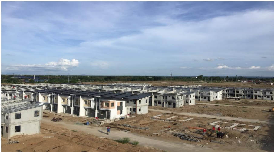
Construction of 450 housing units underway; expected turnover starting Q4
