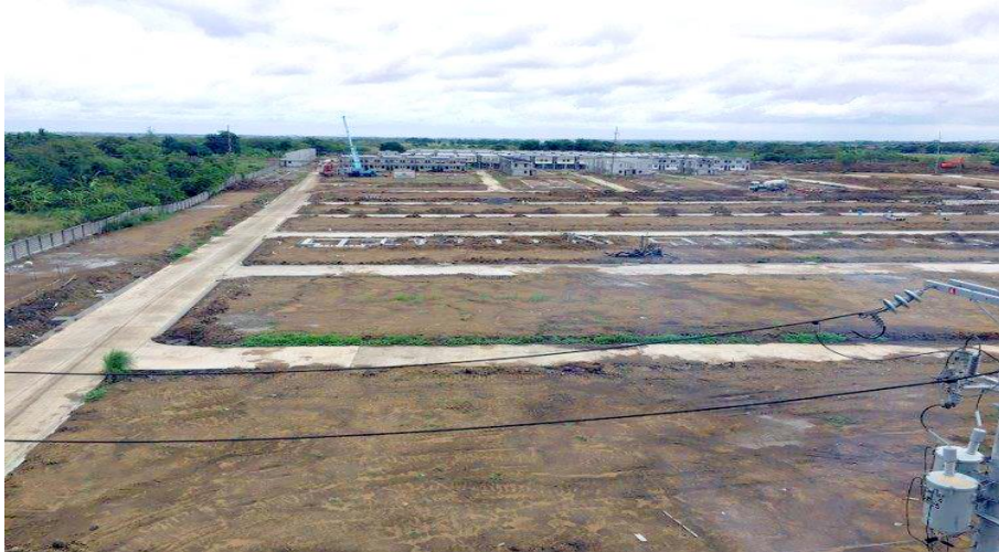
Land Development in full swing, 80% POC in Phase I
