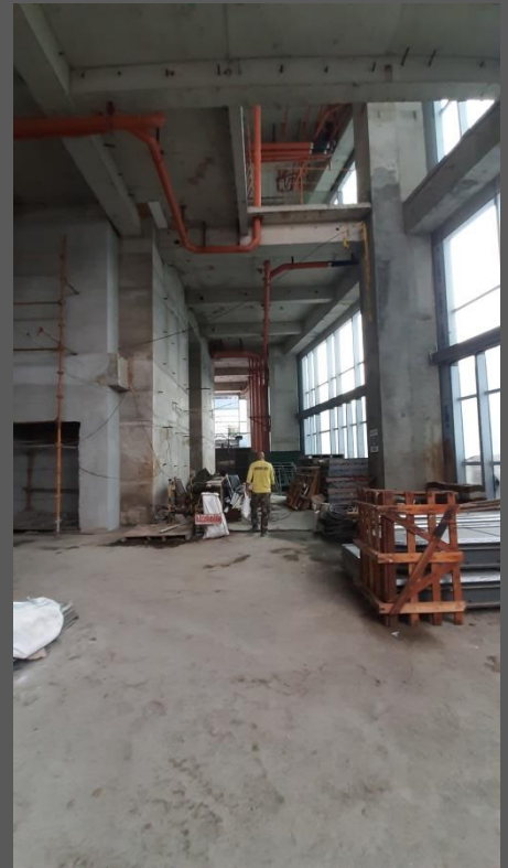
Ground Floor – Retail Area
