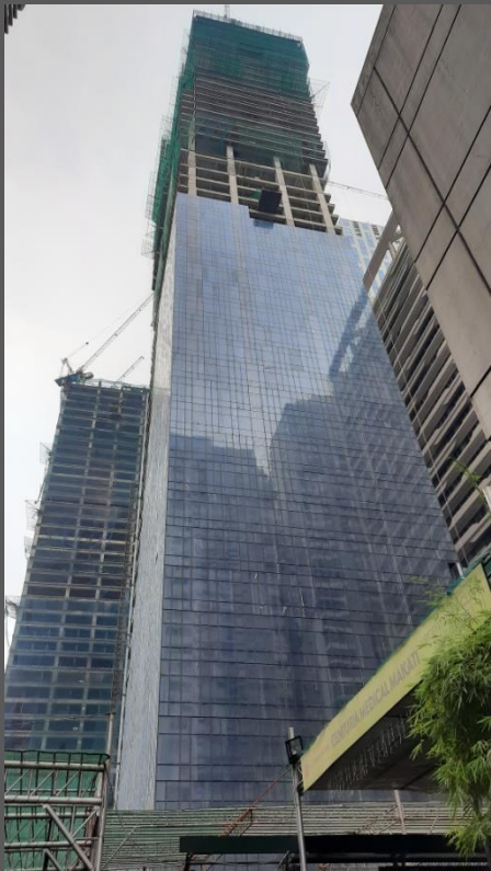
South-East Elevation view from Salamanca Street
