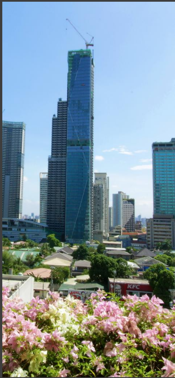
THE TRUMP TOWER CONSTRUCTION
